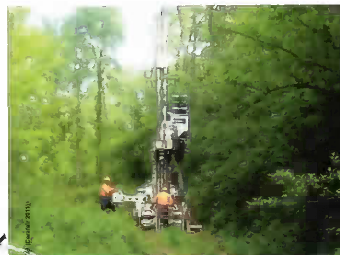
Picture n. 7-8 : borehole with core sampling operations
