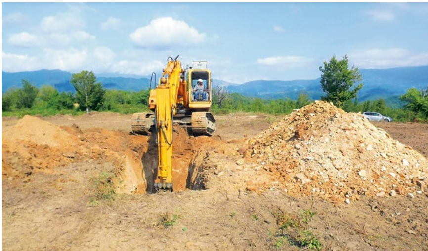
Figure 6 Trench execution with hydraulic excavation for preliminary clay sampling. (© Bertolotti)
